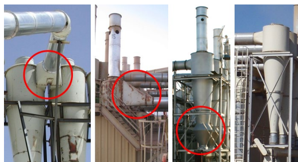
Figure 11. Cyclone design variations for the tested systems (left to right): dual configuration that splits the flow between identical 1D3D cyclones with 2D2D inlets; 1D3D cyclone with an inverted 1D3D inlet; 1D3D cyclone with 2D2D inlet and expansion chamber on the cone; 1D3D cyclone with 2D2D inlet and standard cone.
