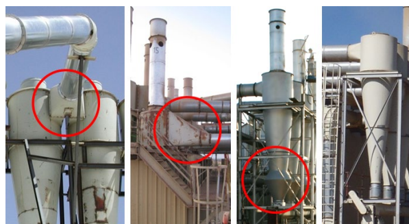
Figure 12. Cyclone design variations for the tested systems (left to right): dual configuration that splits flow between identical 1D3D cyclones with 2D2D inlets; 1D3D cyclone with an inverted 1D3D inlet; 1D3D cyclone with 2D2D inlet and expansion chamber on the cone; 1D3D cyclone with 2D2D inlet and standard cone.
