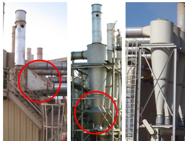
Figure 12. Cyclone design variations for the tested systems (left to right): 1D3D cyclone with an inverted 1D3D inlet; 1D3D cyclone with 2D2D inlet and expansion chamber on the cone; 1D3D cyclone with 2D2D inlet and standard cone.
