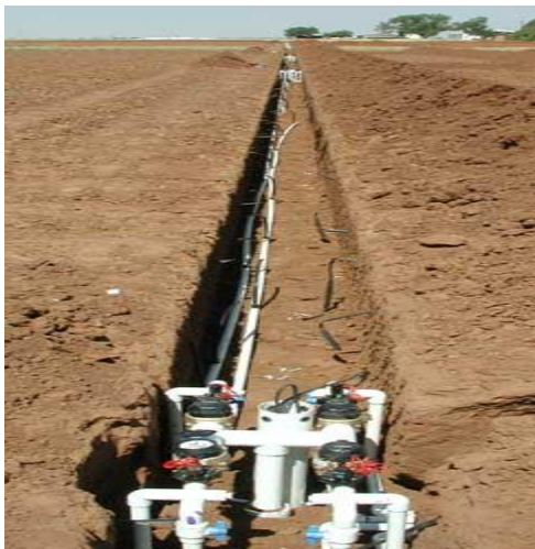
A drip irrigation system was installed at the Munday Research Station in West Texas ahead of cotton planting in 2002.
