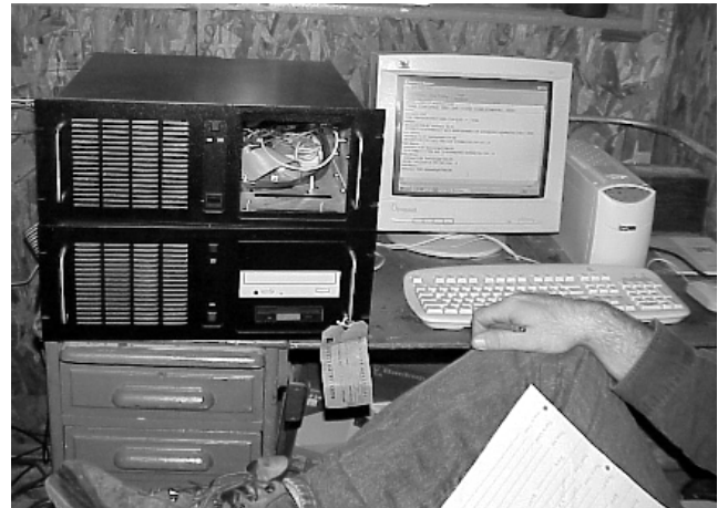
Figure 7. Data logger and cable interface at McClendon, Mann, and Felton Gin.
