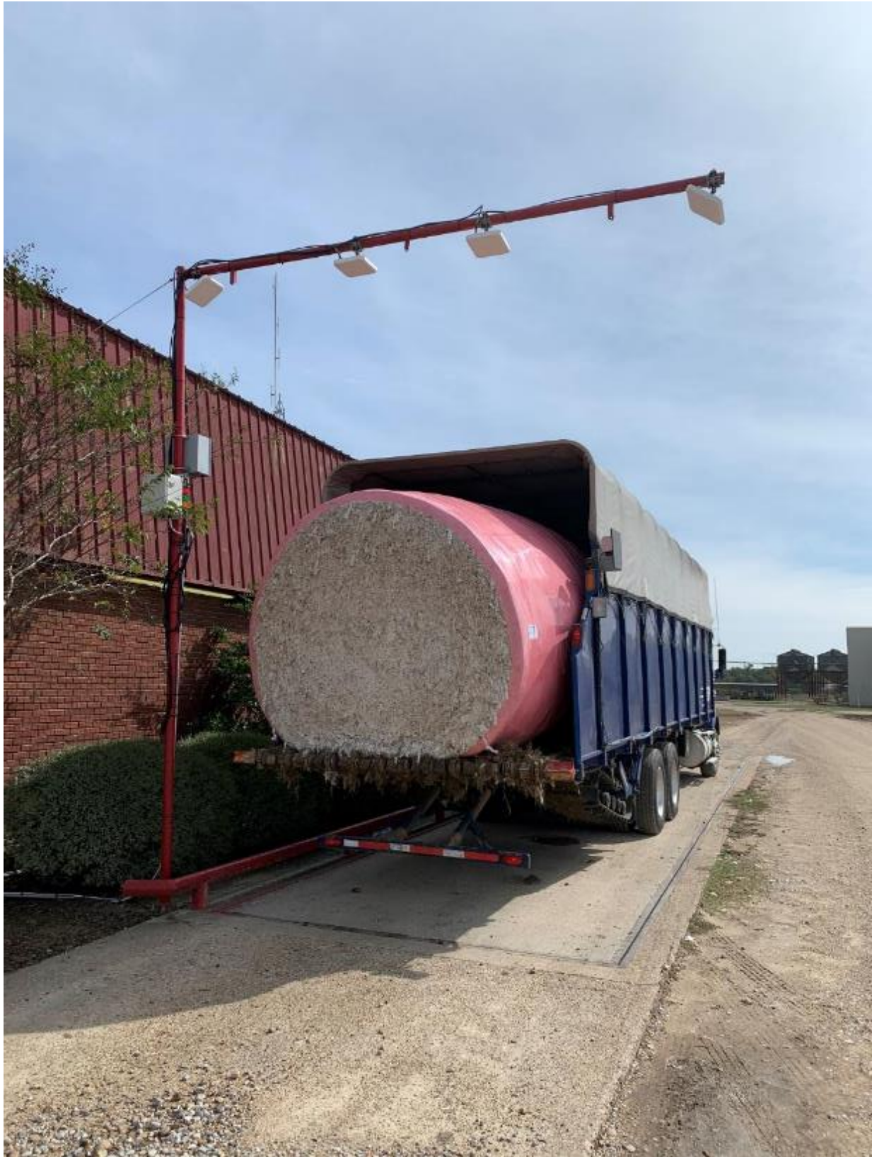
Figure 6. Image of the RFID scanning bridge located at the entrance to the truck scale at Tanner and Co. Gin. Four RFID antennas are positioned on the horizontal top bar while the RFID reader, red/green/amber stack light, and GPIO electronics are mounted to the vertical post.
