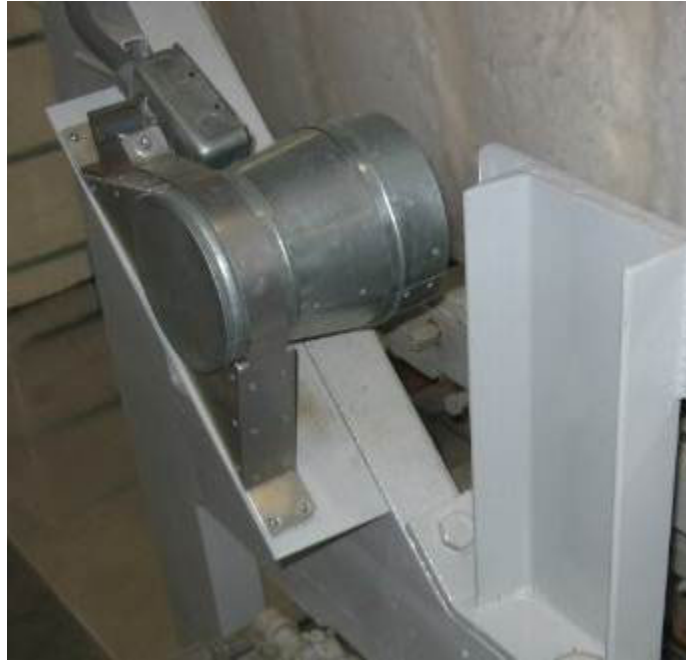
Figure 5. Microwave bale moisture sensor.
