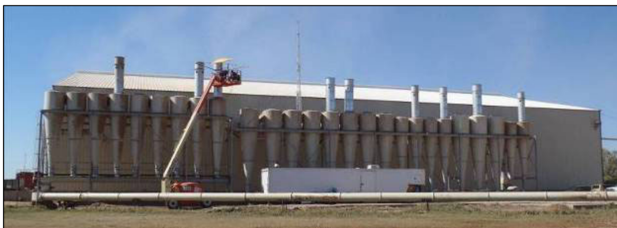
Figure 3. Stack sampling at the West Texas cotton gin.
