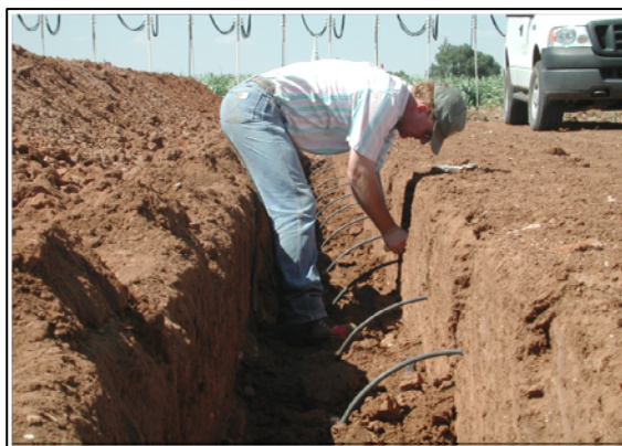
Figure 2. Installation of automated SDI system, Helms Research Farm, Halfway, Texas.
