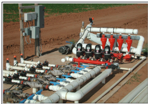
Figure 1. Installation of automated SDI system, Helms Research Farm, Halfway, Texas.
