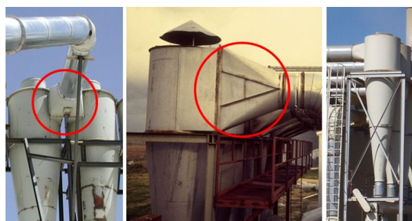
Figure 11. Cyclone design variations for the tested systems (left to right): dual configuration that splits flow between identical 1D3D cyclones with 2D2D inlets; 1D3D cyclone with a center-line 1D3D inlet; 1D3D cyclone with 2D2D inlet and standard cone.
