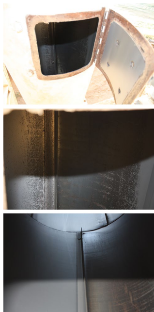
Figure 14. Angle-iron welded to the inside surface of cyclone cone at gin F.
