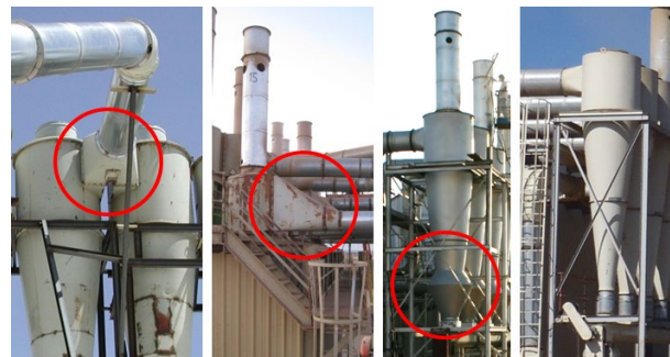
Figure 12. Cyclone design variations for the tested systems (left to right): dual configuration that splits flow between identical 1D3D cyclones with 2D2D inlets; 1D3D cyclone with an inverted 1D3D inlet; 1D3D cyclone with 2D2D inlet and expansion chamber on the cone; 1D3D cyclone with 2D2D inlet and standard cone.
