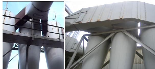
Figure 13. Photographs triple cyclone configurations (left to right): triple cyclone configuration with flow split among three, side-by-side, identical cyclones; triple cyclones in a tandem configuration with flow split among three, one-behind-another, identical cyclones.
