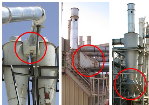
Figure 12. Cyclone design variations for the tested systems (left to right): dual configuration that splits flow between identical 1D3D cyclones with 2D2D inlets; 1D3D cyclone with an inverted 1D3D inlet; and 1D3D cyclone with 2D2D inlet and expansion chamber on the cone.
