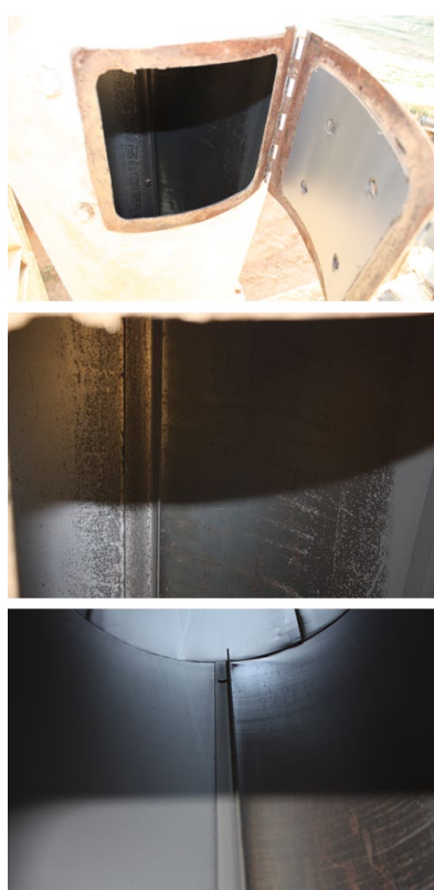
Figure 16. Angle-iron welded to the inside surface of cyclone cone at gin F.
