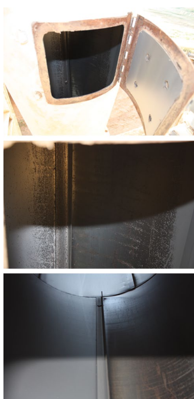
Figure 15. Angle-iron welded to the inside surface of cyclone cone at gin F.
