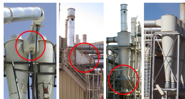
Figure 14. Cyclone design variations for the tested systems (left to right): dual configuration that splits flow between identical 1D3D cyclones with 2D2D inlets; 1D3D cyclone with an inverted 1D3D inlet; 1D3D cyclone with 2D2D inlet and expansion chamber on the cone; 1D3D cyclone with 2D2D inlet and standard cone.
