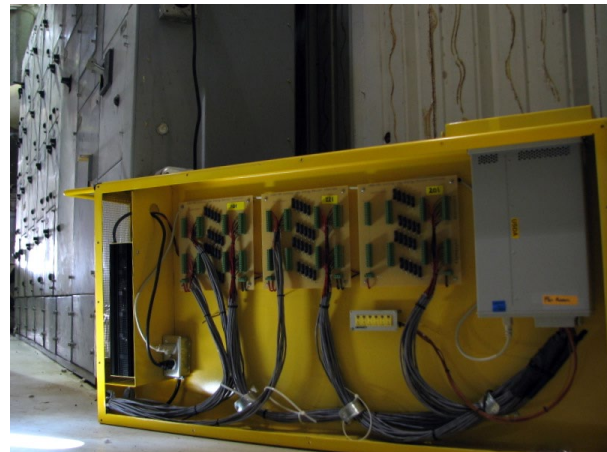
Figure 1. A USDA-ARS data logger (with the cover removed) near a motor control center.
