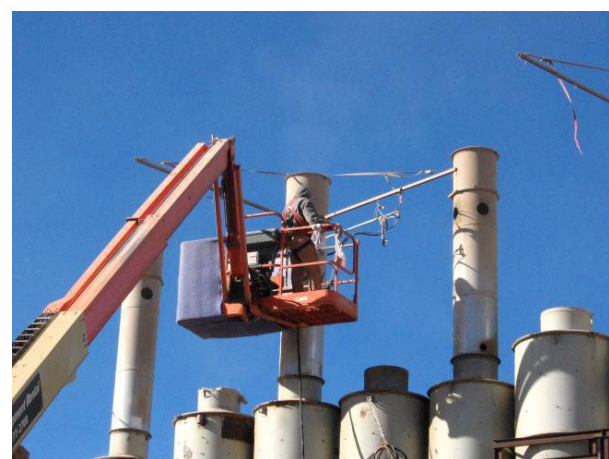
Figure 6. Stack extension installed on cyclone exhausts.
